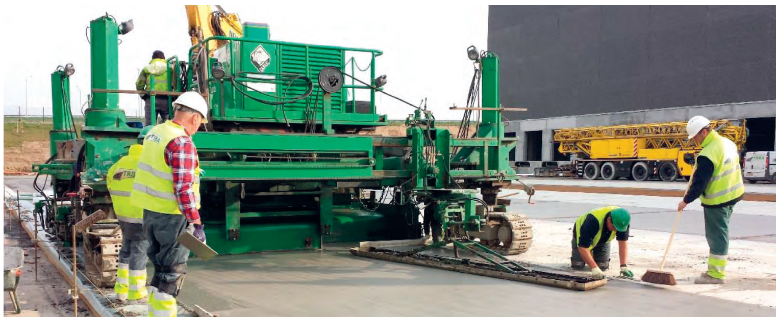
Colruyt Lessines : double lattice reinforced concrete 25 cm thickness
